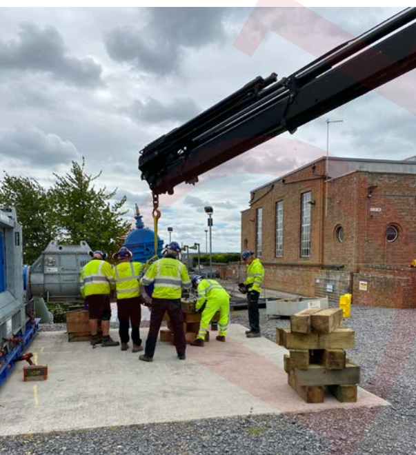
Installing ultra-high volume pumps for taking water from North Drain into the River Brue
